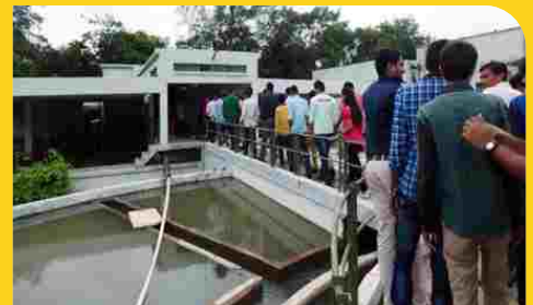
Observing the different components of Aji water treatment plant
