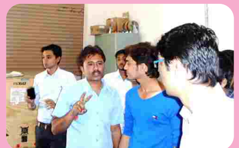
Expert explaining the advantages of Gas Insulated Substation at GIS, Rajkot
