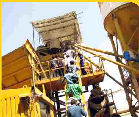
Climbing upstairs with curiosity to watch Mixing process of concrete at UltraTech Cement (Ready Mix Concrete)
